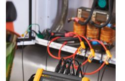
Power Quality monitoring in compliance with EN 50160 at Main Incomer. Power Quality monitoring at UPS input / output The above includes logging of power and P.Q. parameters such as:
